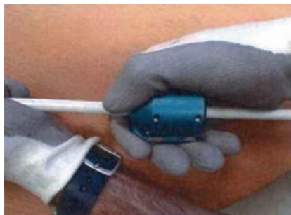
Figure 1 : opening a CU cable
